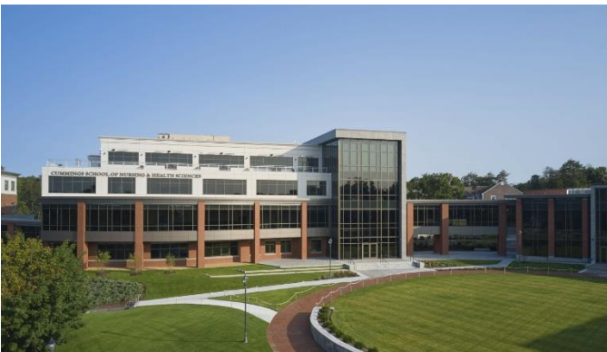
Cummings School of Nursing & Health Sciences Endicott College, Beverly, MA Windover Construction
